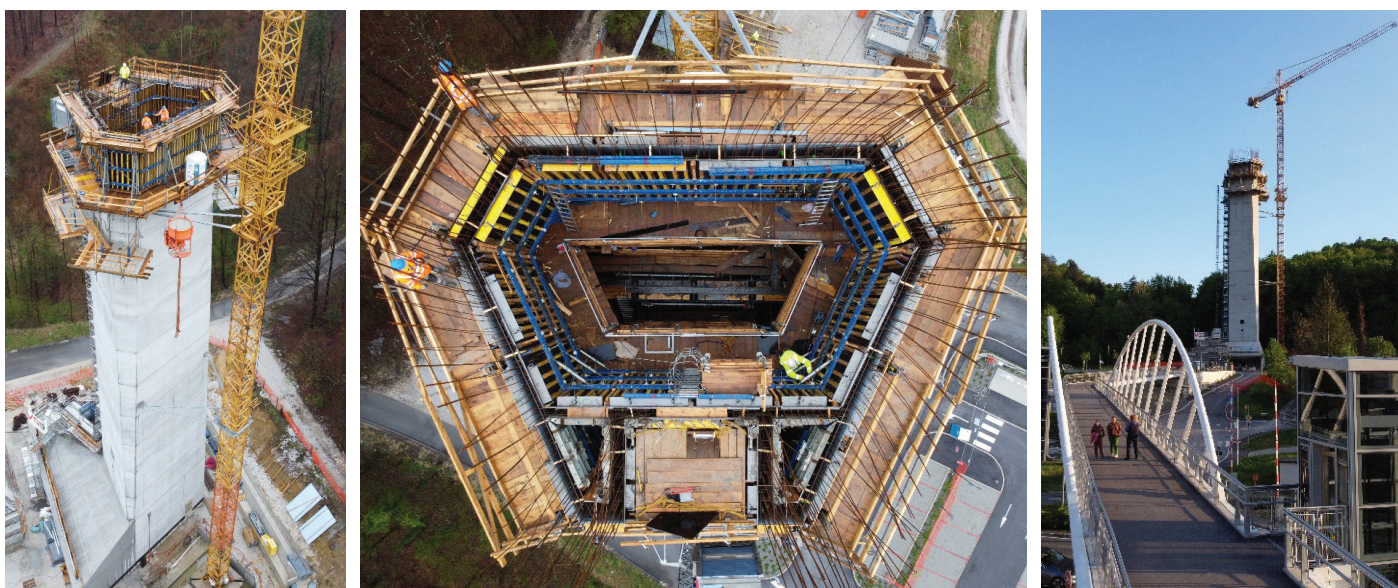
Slike 14, 15, 16. Betoniranje 13. segmenta stebra, h = 50,05 m (14. 4. 2023).
